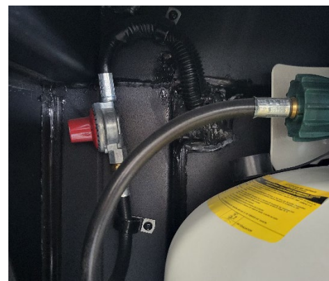
Figure 28. Step down propane regulator for long hose lengths, dropping pressure from tank levels to 30 psi.
