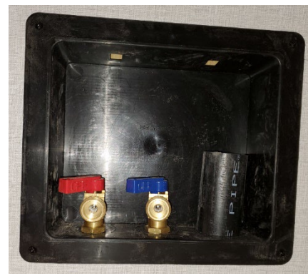
Figure 139. Washer connections and drain.
